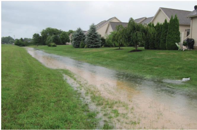
Figure 3c. Not all lawns drain into storm sewer inlets. Many drain into grass swales or roadside ditches that also drain into local waterways. (Andy Yencha)
