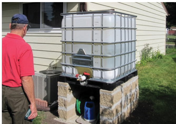
Figure 28b. Large vessel used for lawn or garden irrigation. (Andy Yencha)
