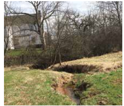
Continual erosion has caused the need to restore the streambank along the East Branch of the Perkiomen Creek that winds through Jacob Reiff Park.
