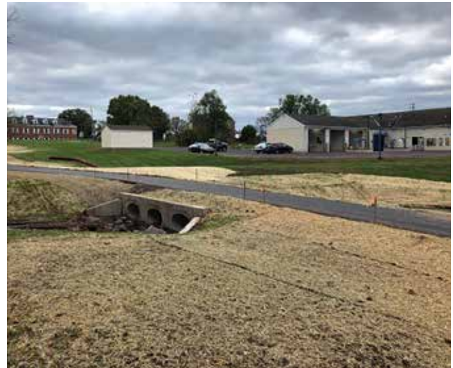
Overview of completed path with Clemens Road to the left
