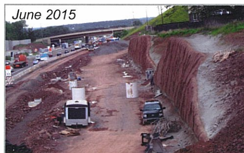
E-ZPass Auxiliary Ramp F-1. Left: Rough graded outline of the new ramp. Right: New ramp with completed concrete pavement, traffic barriers, and E-ZPass gantries.
