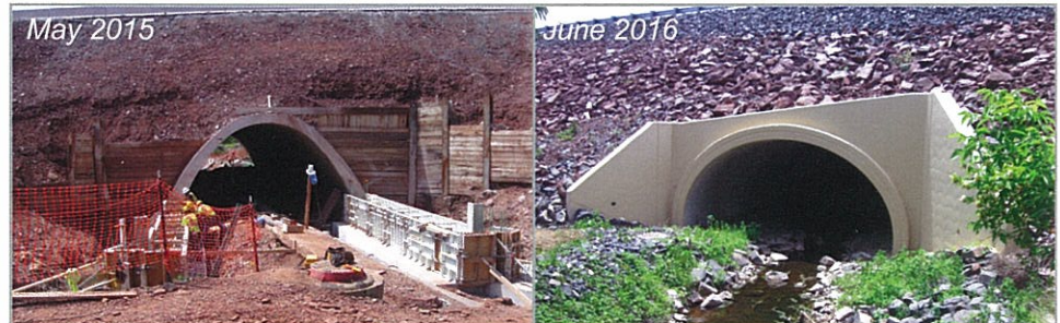
Arch Culvert. Left: Forming of the new arch culvert. Right: Fully-constructed new culvert.
